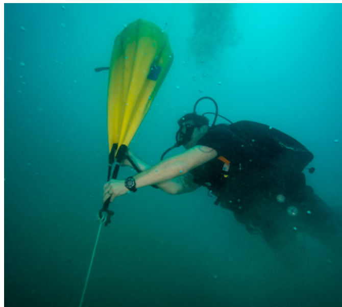
Explosive ordnance disposal diver fills a lift balloon attached to a simulated bottom mine in the Mediterranean Sea during an exercise. When underwater explosive ordnance is deemed safe to move, removal is a clearance method that minimizes environmental impact. Removal can be done also with a remotely operated vehicle or a salvage vessel crane. © U.S. Naval Forces Central Command/U.S. Fifth Fleet
